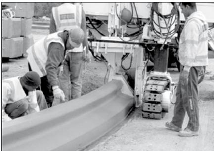
**Part of the slipformed high containment kerb constructed on a tight radius**
