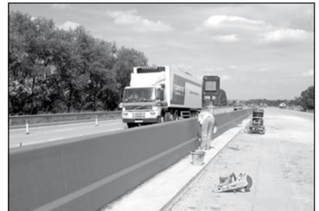
Construction of the new concrete step barrier began in June on the M62 motorway near Hull in East Yorkshire. These works represent the first implementation of the Highways Agency instruction to provide higher performance in-situ concrete safety barrier rather than steel barrier along all motorway medians.
