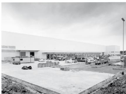
**Traditional construction of a concrete hardstanding alongside fast track building construction**
