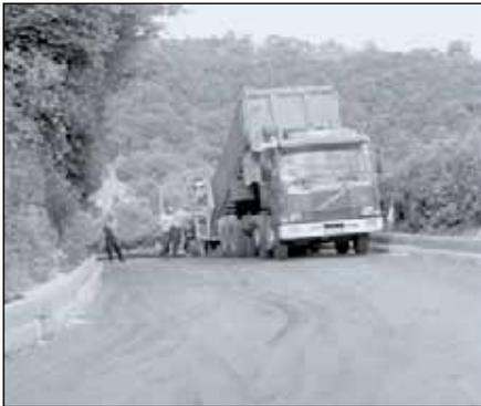
**Reconstruction of the A52 in Staffordshire, where planings used as the aggregate were relaid after stabilisation off-site with lime and PFA.**
